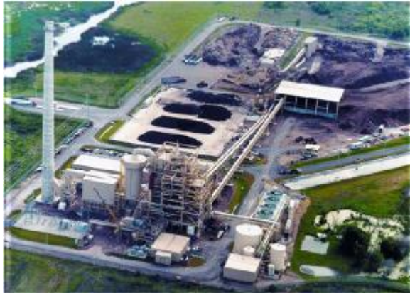
Ridge Generating Station 40MW Wood Waste and Tire-Fueled Power Plant Lakeland, Florida
