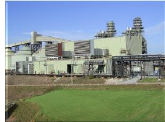
Aughinish 150MW Combined Heat and Power Plant Askeaton, Ireland
