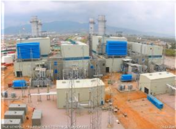
Skikda 820MW Combined Cycle Power Plant Skikda, Algeria
