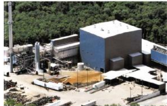
Sterling 26MW Tire-Fueled Power Plant Sterling, Connecticut
