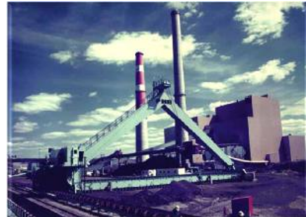
Battle River 675MW Thermal Generating Station Alberta, Canada
