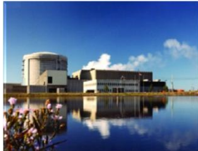
Point Lepreau Nuclear Generating Station New Brunswick, Canada
