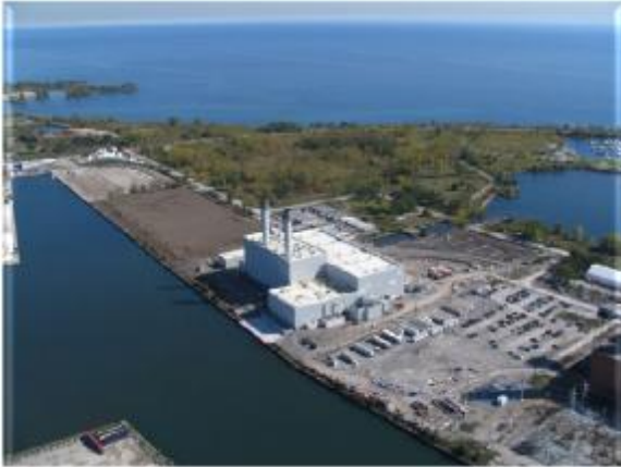
Portlands Energy Centre 550MW Combined Cycle Power Plant Toronto, Ontario
