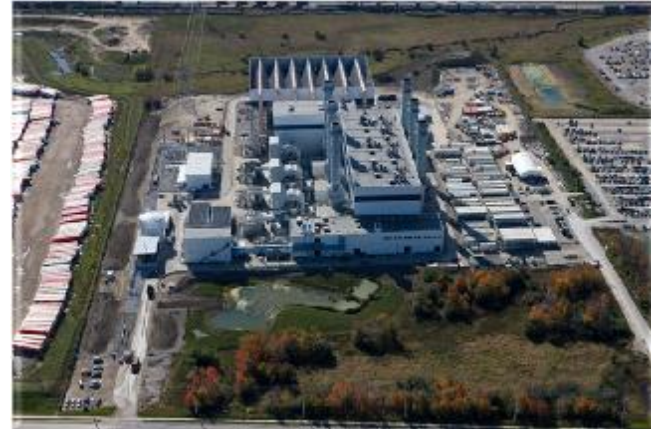
Goreway Station 880MW Combined Cycle Power Plant Brampton, Ontario
