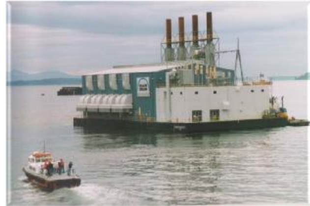
Corinto 70.5MW Barge Mounted Floating Power Plant Nicaragua
