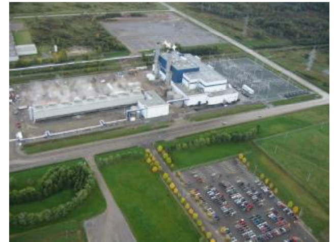
Becancour Combined Cycle Cogeneration Project Becancour, Quebec, Canada
