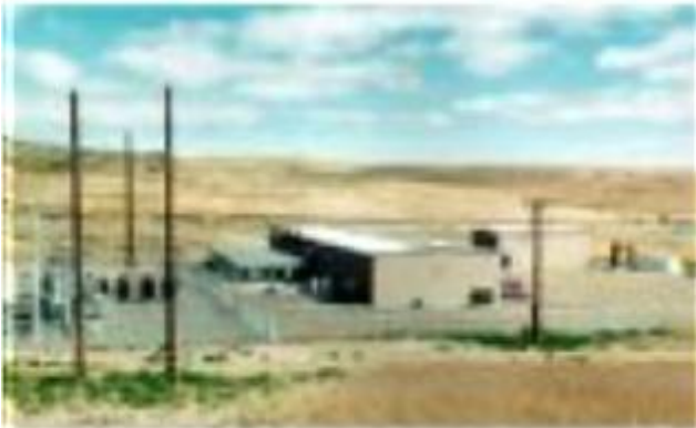
10.5MW Landfill Gas Power Plant Roosevelt, Washington
