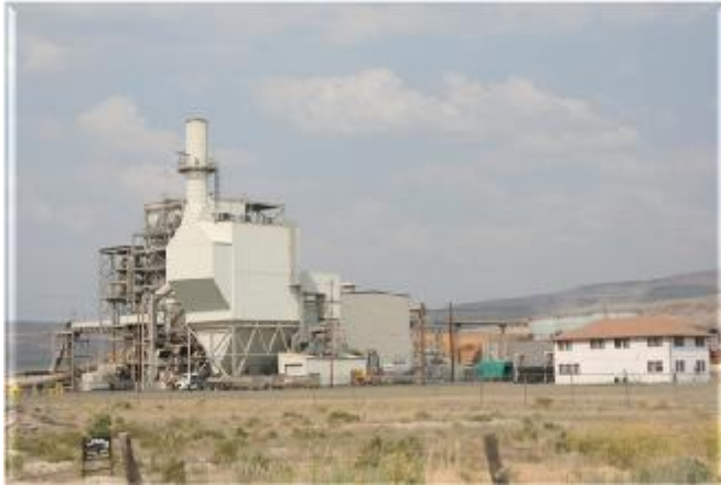
Honey Lake 30MW Wood-Fired and Geothermal Power Plant Wendel, California
