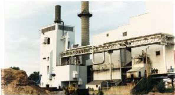
Burlington 200TPD Biomass Gasification Facility Burlington, Vermont
