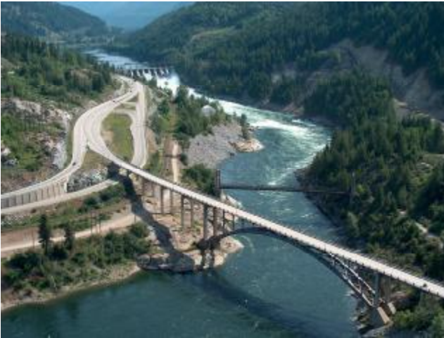
Brilliant Expansion Project British Columbia, Canada
