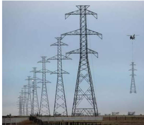
AltaLink Southwest Development Project Alberta, Canada
