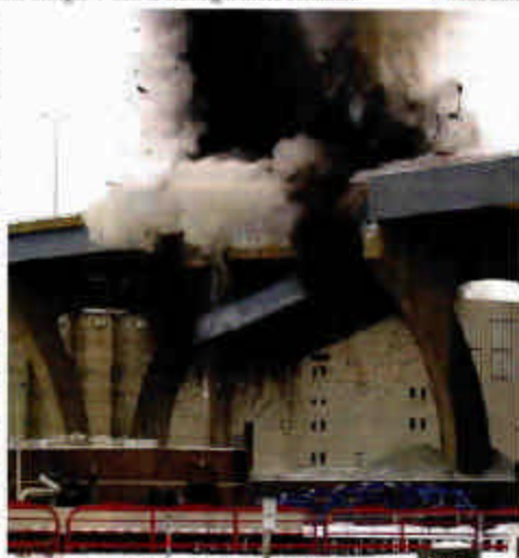
SEQUENCED FALL Bridge span was dropped in three segments.
