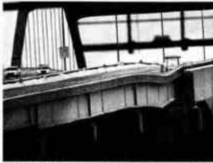
BUCKLED Girder failure caused 4-ft dip in bridge, says state.
