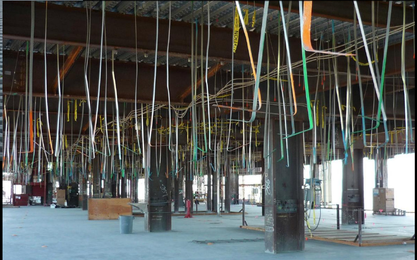
Palomar Medical Center West – CO Architects
