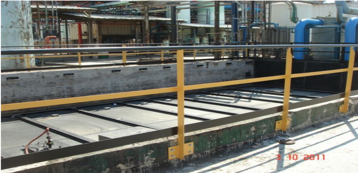
Below Grade API Units
