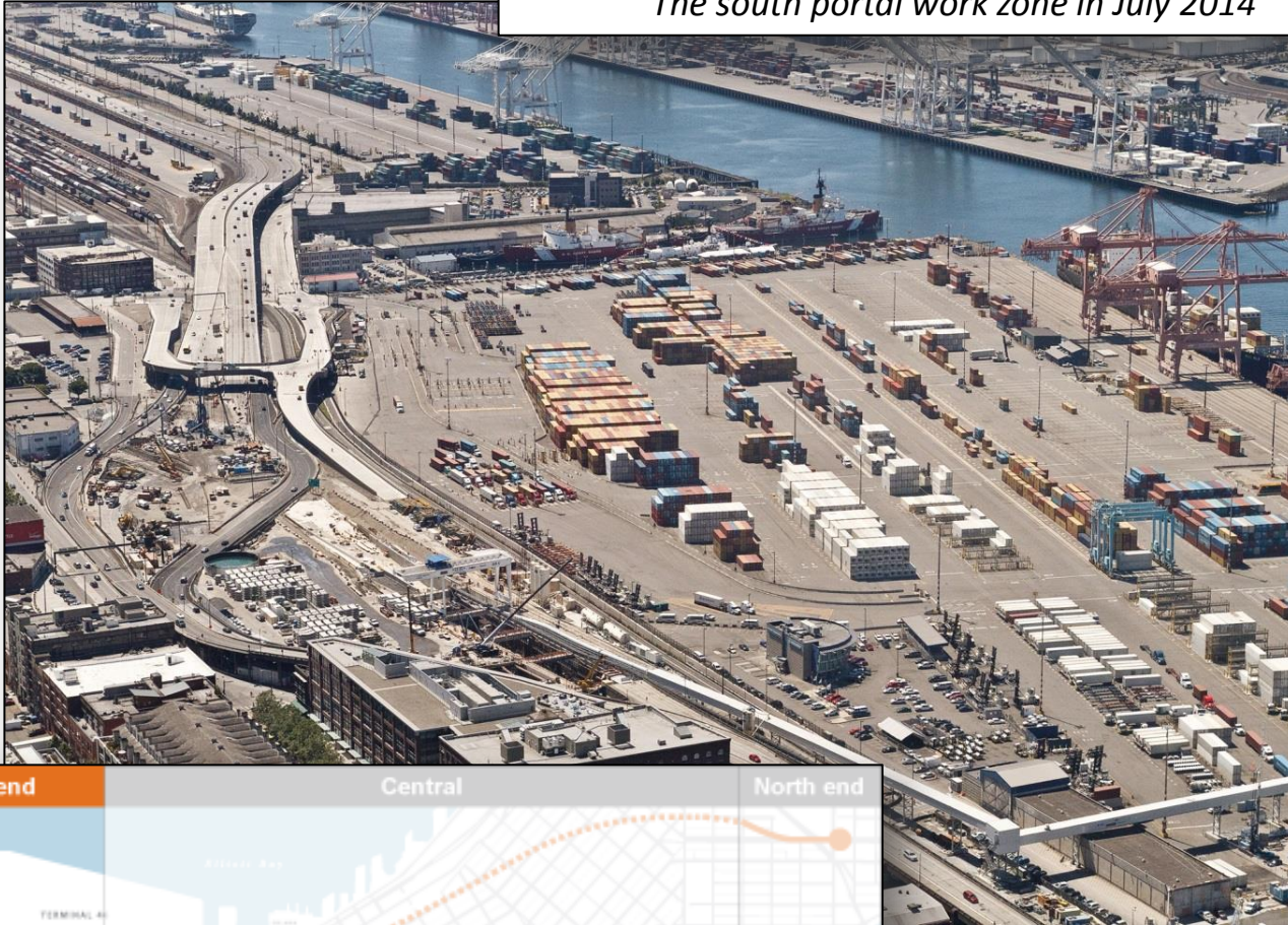
The south portal work zone in July 2014
