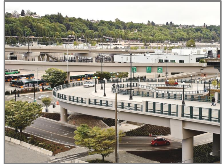
SR 519 Intermodal Access Project.
