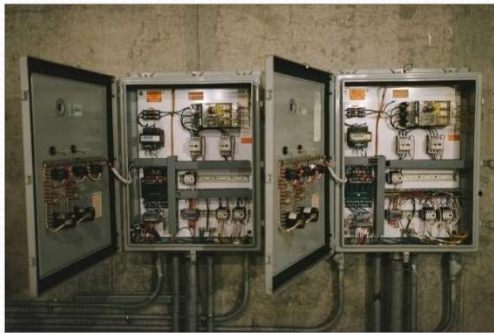
Equipment Control Panels – Cleaned, inspected, and ready for repair/replacement
