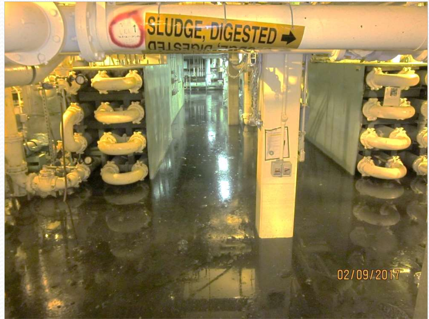
Flooded equipment galleries
