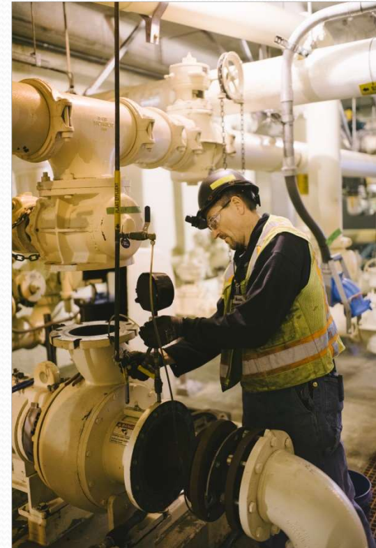
Pumps being repaired
