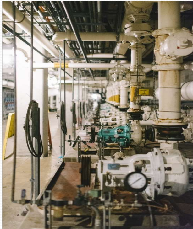
Gravity Belt Thickener Feed Pumps - Ready for replacement motors
